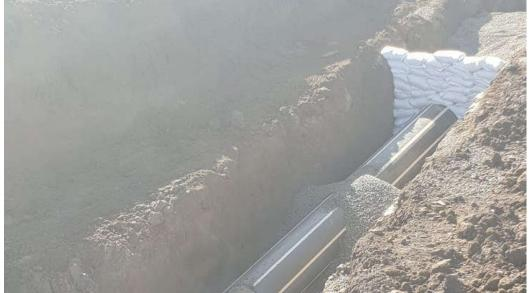
Civcorp was engaged on short notice to lay multiple sewer rising mains and gravity mains as part of the Flagstone to Cedar Grove Waste Water Treatment Plant Conveyance System. Civcorp's ongoing relationship with Logan Water Alliance and experience in pipelaying and HDPE pipe were key in ensuring the project stayed on schedule and on budget.
